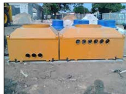
For operational and maintenance reasons, there are no valves inside the MBOX6 manifolds. Each dispenser is equipped with a multifunction under pump valve and a manual shut-off valve is installed on the tank manway lid to close the suction line when required. These components are optionally available.
